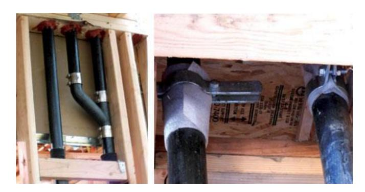
Plumbing joints with pipes nested in joint to allow for vertical movement of structure. Photo courtesy of WoodWorks
